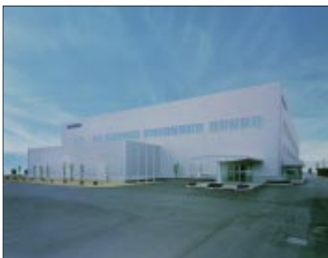
New "FC-1" production facility for FC-3000
